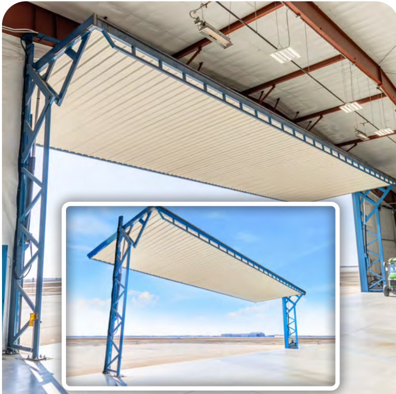
Free-standing structure: the door and its loads stay within their own frame
