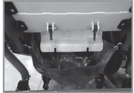
Cleanout Chute installed
