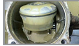
Oil After Diaphragm Rupture
