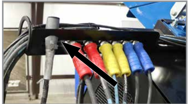
Light Harness Storage Location
